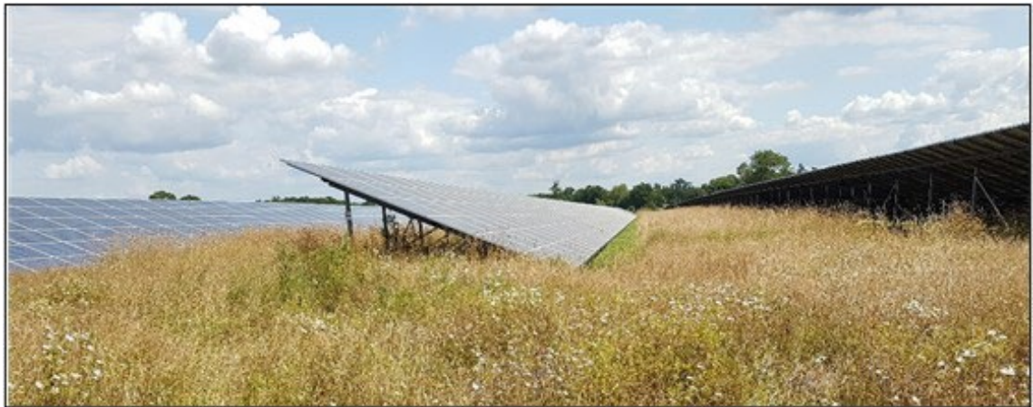
Figure 4.3: Sites where a “Shade Cut” has been employed during the growing season to prevent shading of panels, but allow flowering meadow elsewhere
